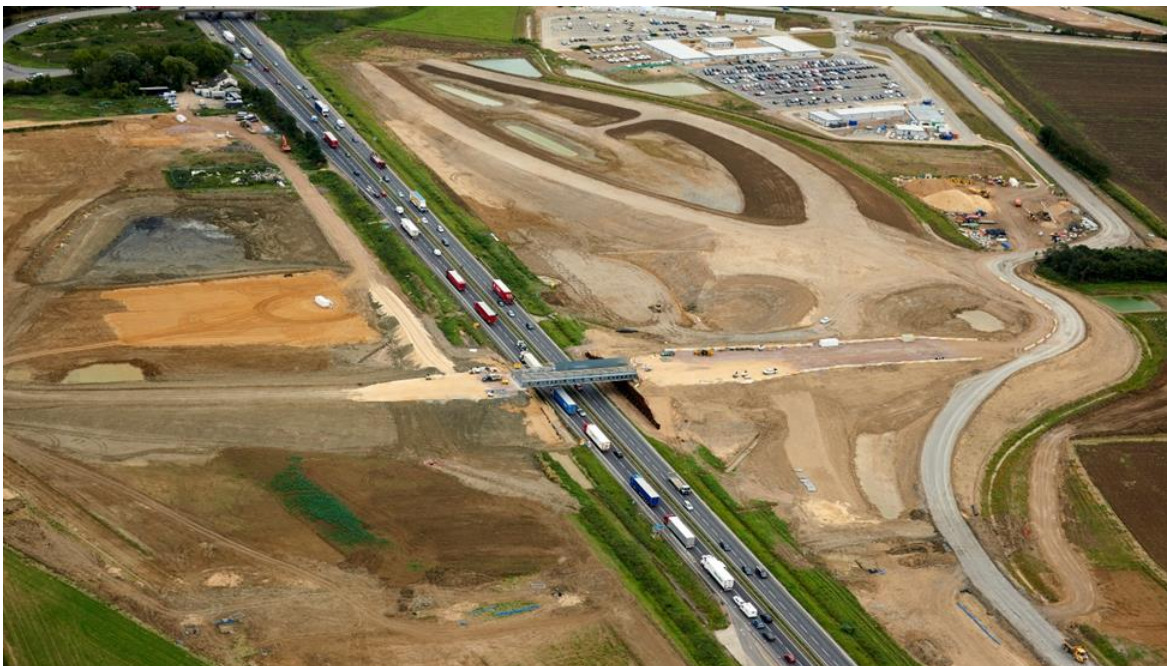
Bailey Bridge over the A14 at Swavesey
