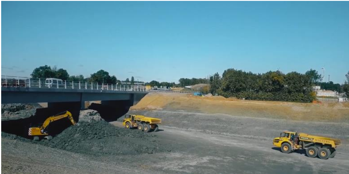
The New Ermine Street Bridge
